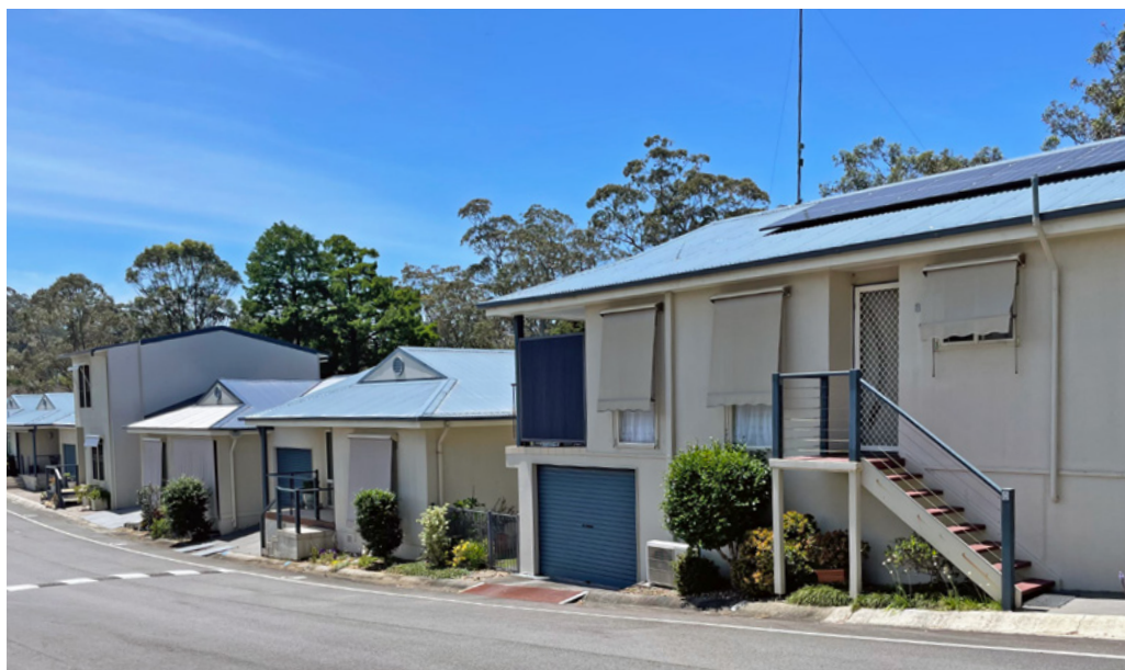
Solar panels on a roof at Terrigal Sands land lease community.
